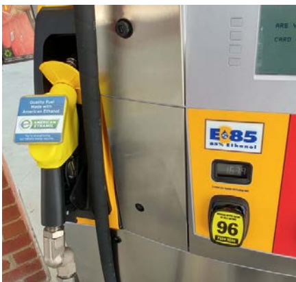
E85 Flex Fuel Dispenser at a Harris Teeter station with ethanol and octane information
