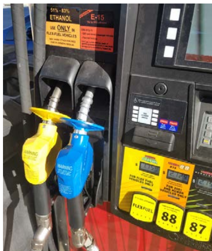
E85+E15 Blender Pump at a Sheetz station
