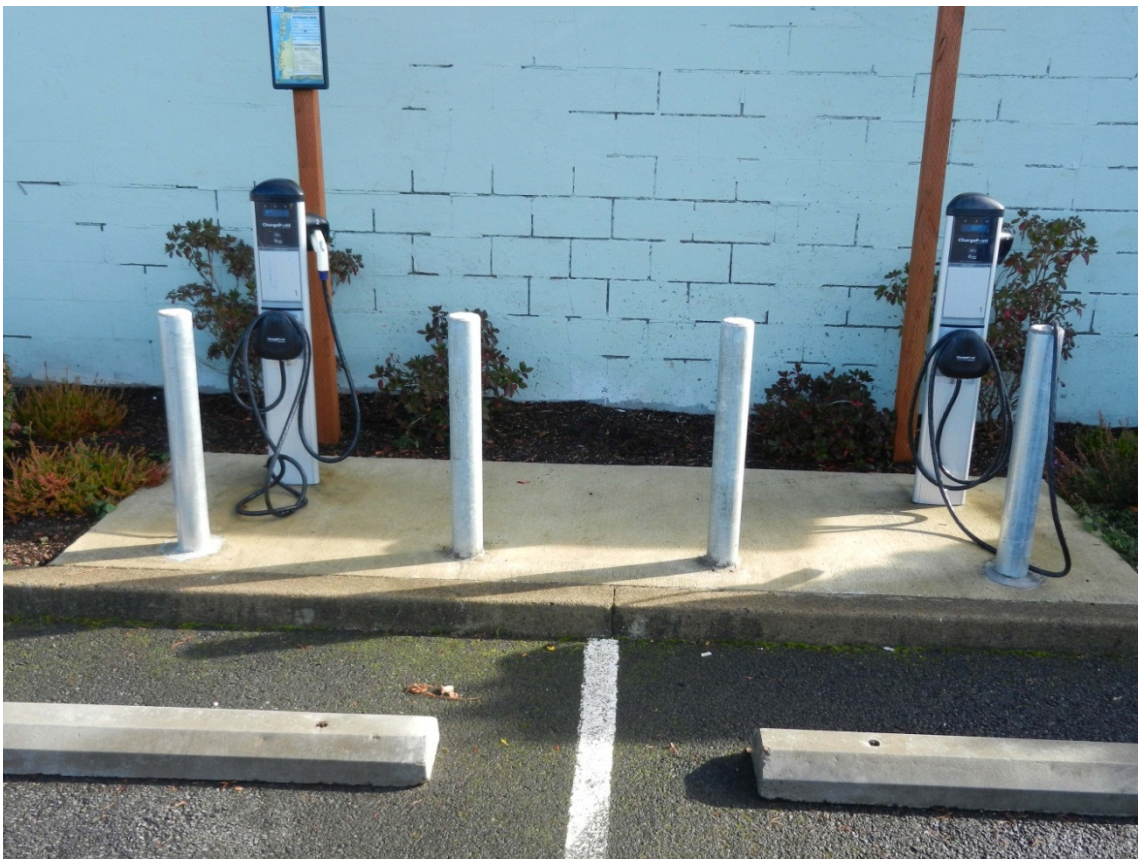
FIGURE 7: BOLLARDS, WHEEL STOPS, AND CURB BLOCK ACCESS
